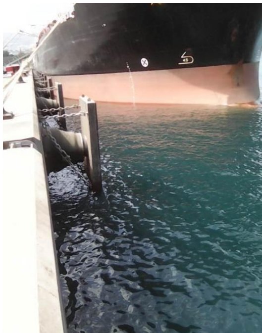
Figure 25. (Copyright Cedre). Illustration showing possible booming effect “of fixed fender system positioned alongside a ship's hull.
